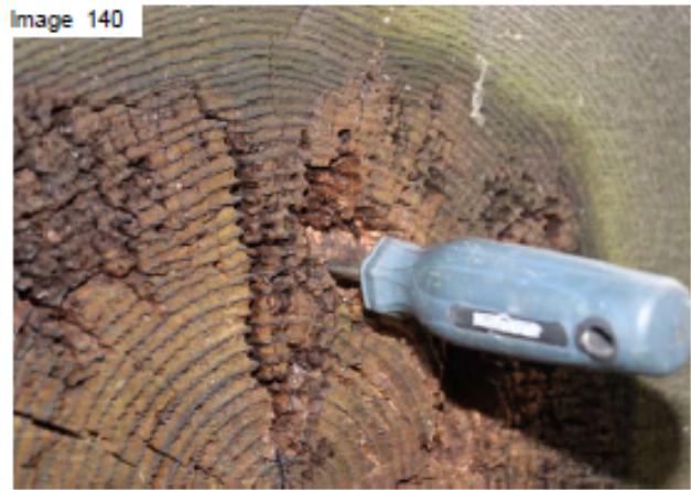
East pier north cross cap decay
