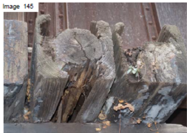
East abutment timber shim decay
