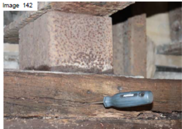
East pier north cross cap decay
