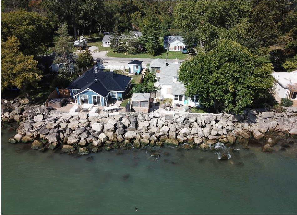
Figure 2: Shore parallel armour stone structures along Pulley Road.
