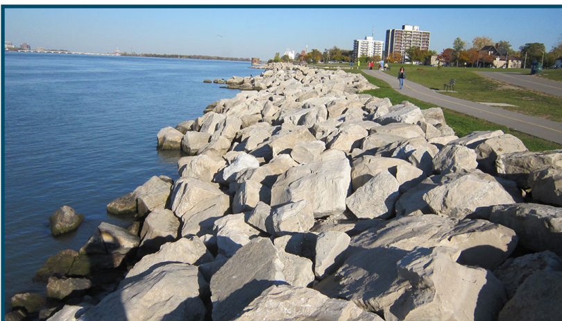
RTB Revetment (between Glengarry Avenue and Louis Avenue)
