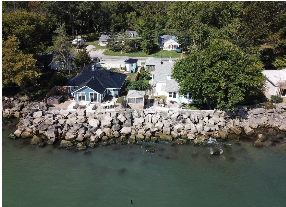
Figure 2: Shore parallel armour stone structures along Pulley Road.
