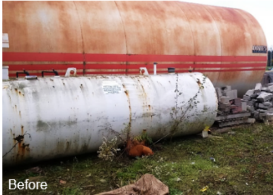
Example of above-grade fuel oil storage tank
