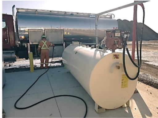
Example of above-grade fuel oil storage tank
